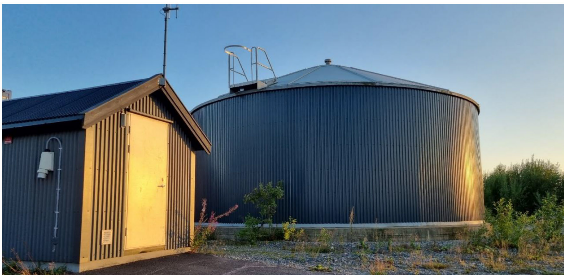
Figur 14 HB Blakstadheia under etablering (november 2012)
